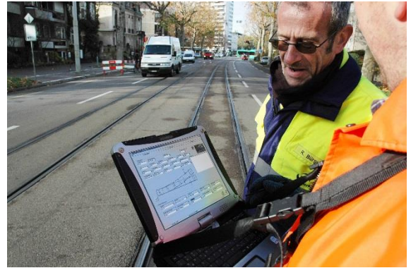
Figure 10: Main inspection of the Basel network supported by MR.pro®. Photo: Peter Binetti (BVB Basel)
