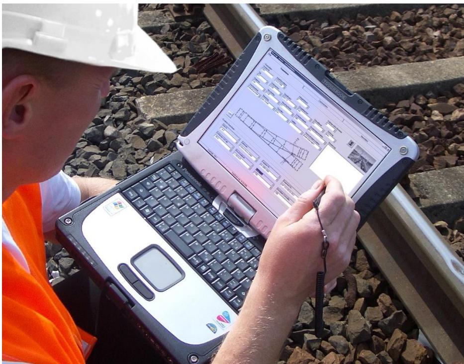
Figure 5 Visual check as well as technical inspection of a turnout with MR.pro®
